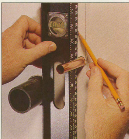
The supply pipes and drain of a kitchen sink are marked on the wall with the aid of a carpenter's level (above). The precise location of the fixtures will then be marked onto vertical and horizontal site story poles before being transferred to the story poles for the sink cabinet itself.
